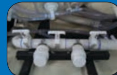
Heat Pump / Gas Heater Connections
